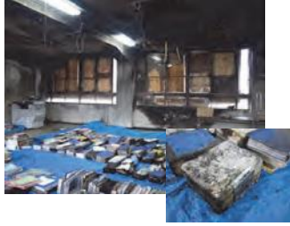
Kamaishi City Hall, which suffered a second disaster due to fire after the Great East Japan Earthquake
